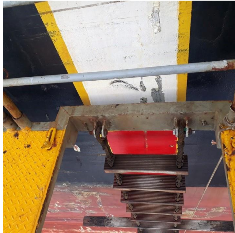
Non-compliant embarkation platform (courtesy of #dangeroussladders)
