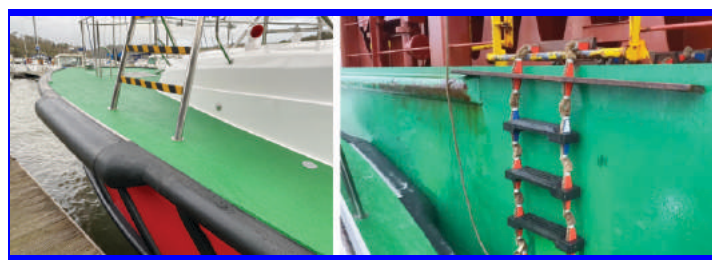
Above, Safehaven's Sacrificial shoulder fender and the gap it creates for the ships pilot boarding ladder
