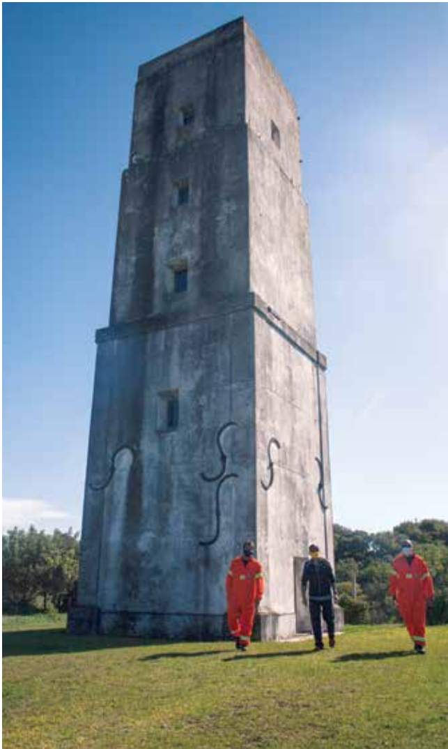
THE OLD PILOTAGE WATCHTOWER
